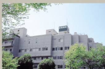
Yokohama Shin-midori General Hospital
